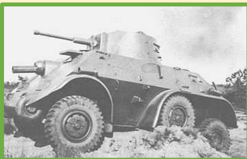
(Above Left, Centre) The M39 under going trials, the rear gunner operated the rear driving controls. (Right) M39 in German service.
