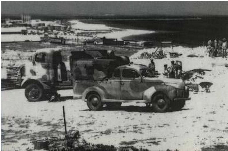
Construction at Leighton Battery on Buckland Hill. The Fremantle Harbour North Mole is visible in the background.
