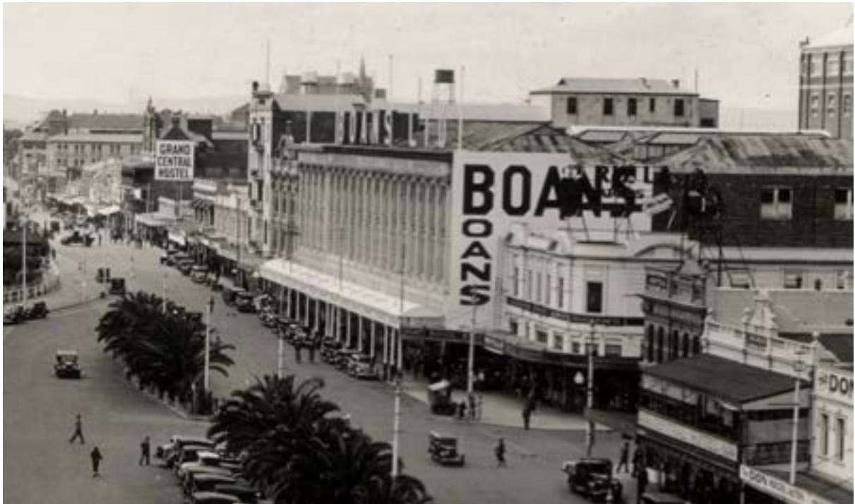
Boans Building Wellington Street circa 1936
