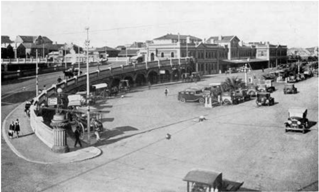
Horseshoe Bridge and Perth Railway station
