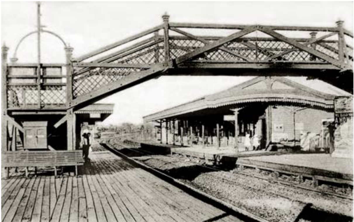
Subiaco railway station c1935
